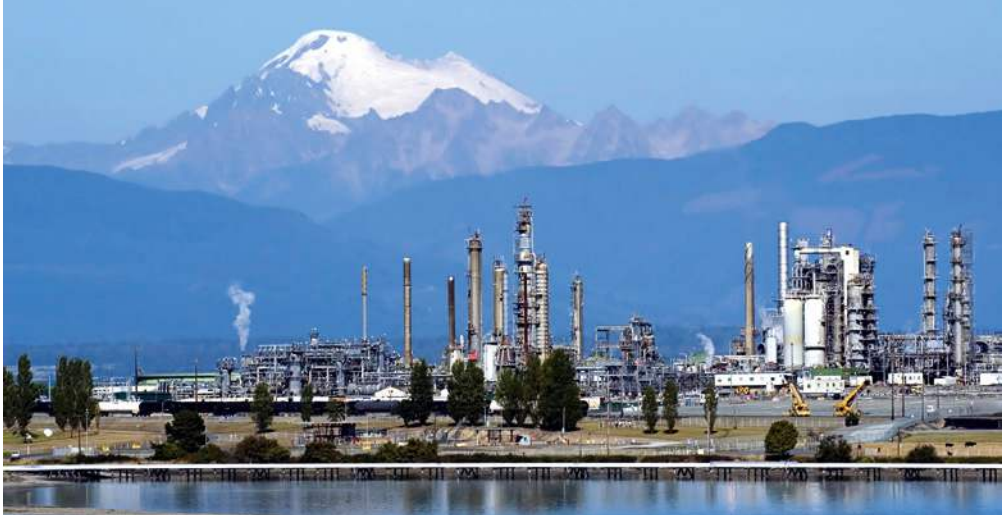
Anacortes Oil Refinery, Washington State, USA
