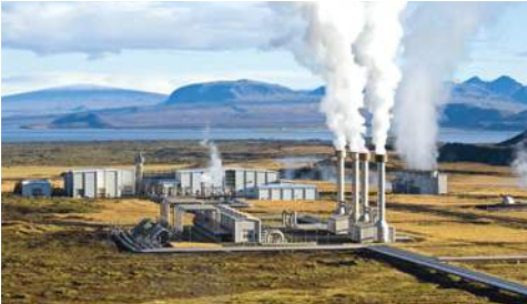
Nesjavillir geothermal plant in Thingvellir, Iceland
