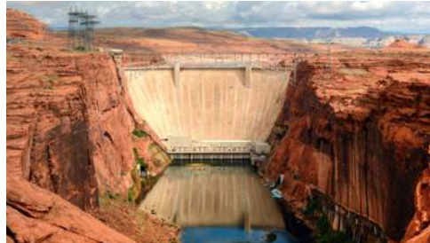
Glen Canyon Dam hydroelectric plant in Arizona, USA
